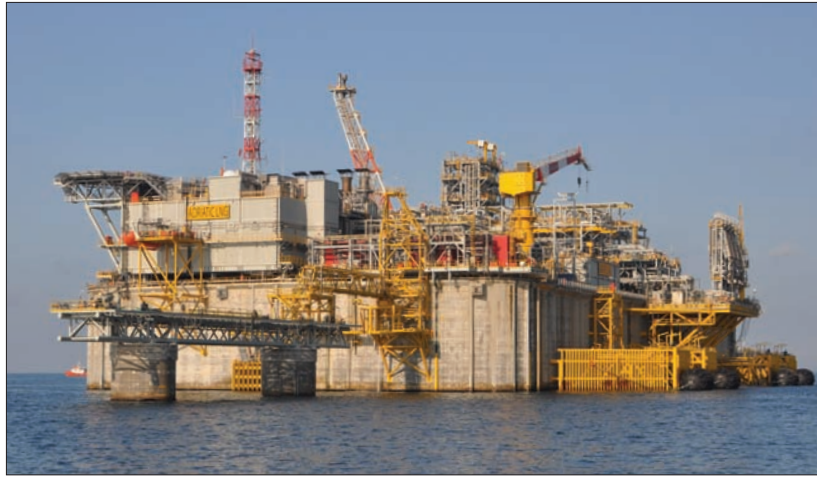
The Adriatic LNG Terminal is the world's only fixed offshore LNG storage and regasification terminal.
