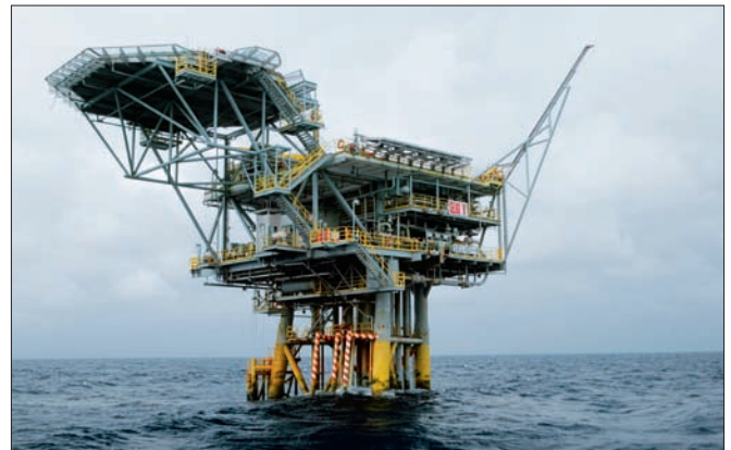
One of the latest-generation satellite platforms at the Telok and Damar fields in Malaysia.
