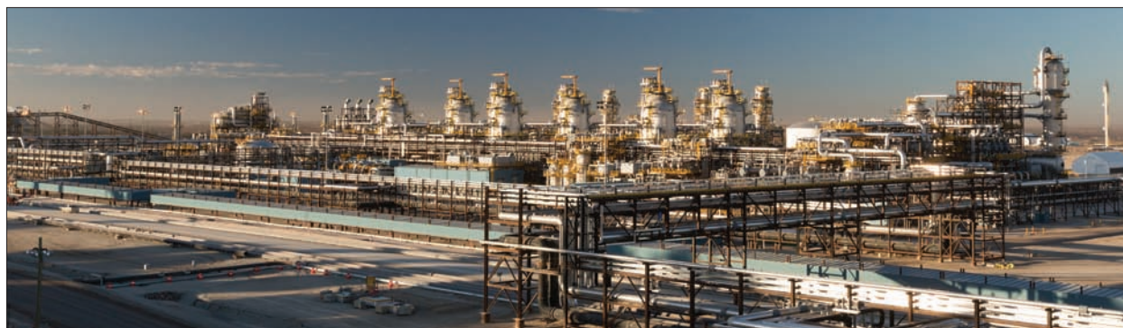
The Kearsarge Expansion Project was completed in 2015, doubling bitumen production capacity.
